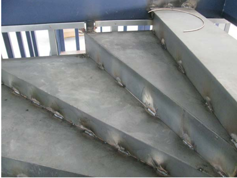
Welded Stair Case
