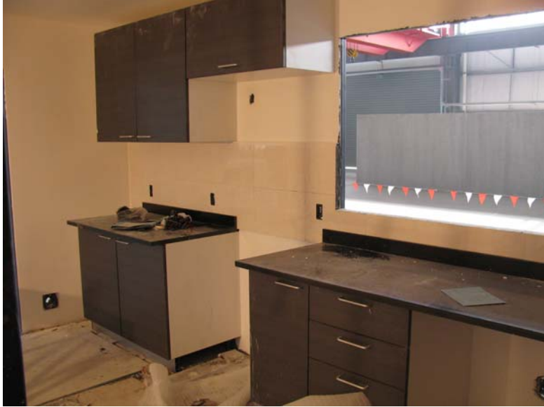
Kitchen Part Finished
