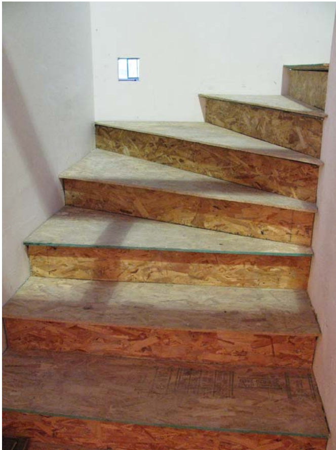
Stairs and Drywall Part Finished.
