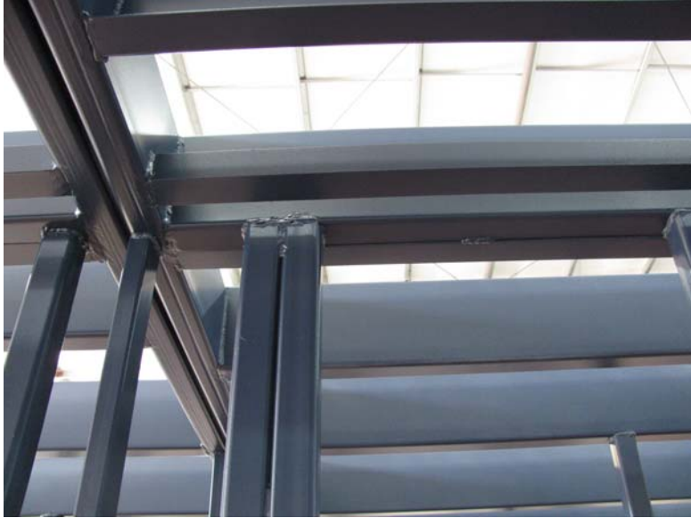
Welded Heavy Gauge Steel Frame
